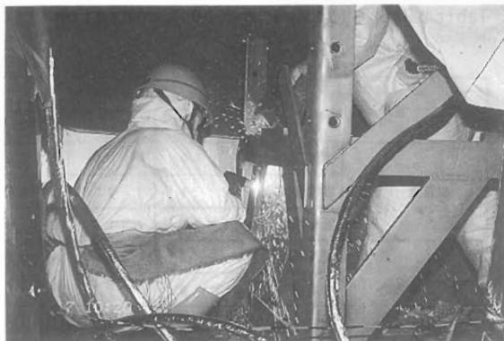
Photo1 Cutting work on core components
