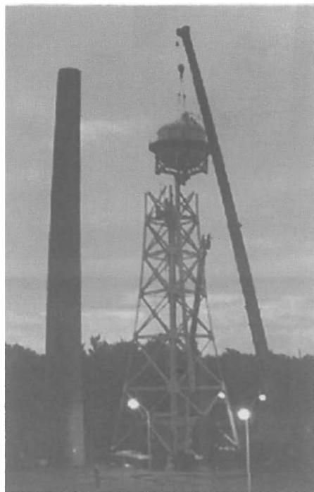
Photo 5 Dismantle of overhead tank
