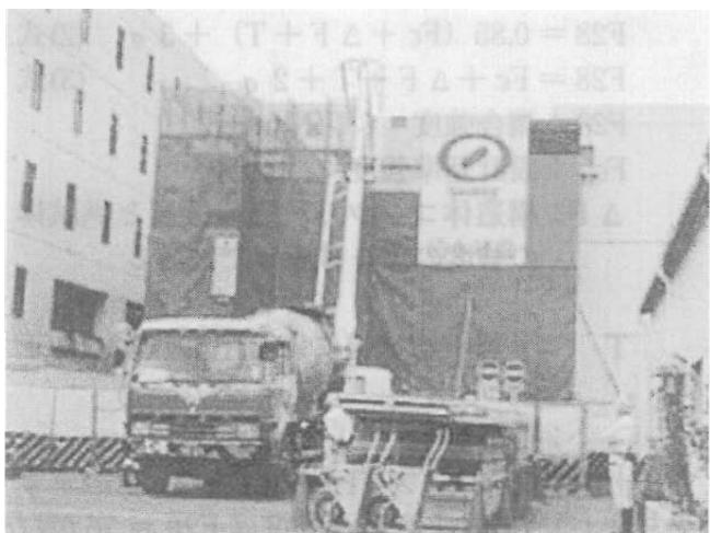
Photo 7 Concrete Placing
